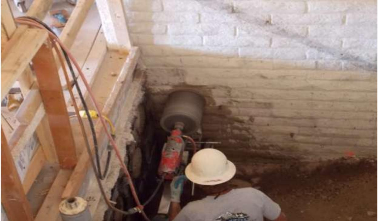
Core Drilling for Heating and Cooling Pipe Pathway
