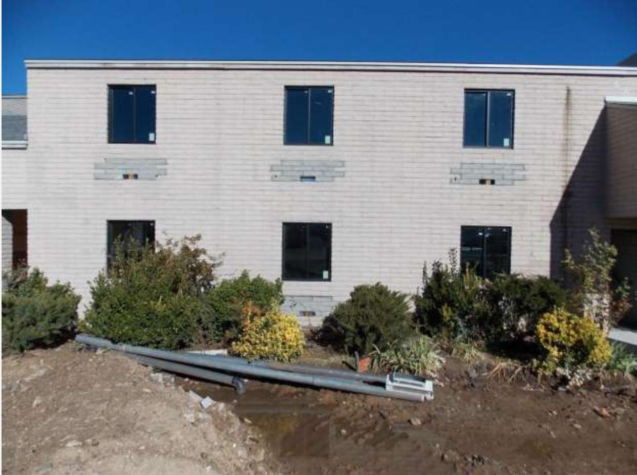
New Windows and Masonry Work after Removal of Room Heating/Cooling Units
